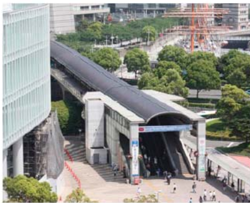
Figure 26: Moving Walkway PV System in Yokohama 78
